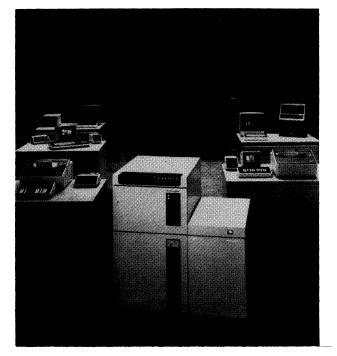
Burroughs CP 9582 communications processor system (foreground center), shown here with various related Burroughs terminals, serves as a financial controller system, manufacturing data collection system, and general purpose terminal control and distributed processing system. The CP 9582 performs line protocols, message handling, and screen formatting functions for the terminals. It then passes the edited transactions to a Burroughs or non-Burroughs computer for processing.
